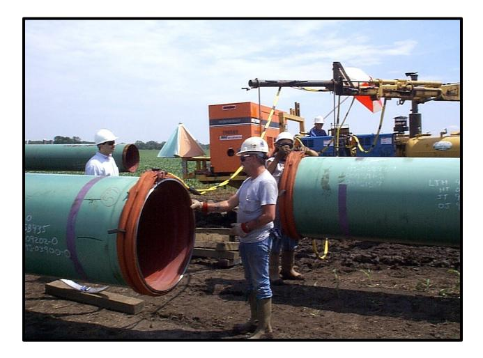
Transmission pipeline construction projects usually require preheat for welding. These 36" diameter pipe ends are being heated with the originally designed induction heating blankets. This led to the addition of Kevlar sleeves for protection. Workers mark the ID with a temperature indicator and give a "thumbs up" to the tractor operator. He then shuts the induction power sources down via a remote on/off control.
