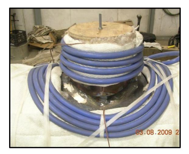
Coil flexibility is important to be able to accommodate various geometries. In this application, a short pipe segment is being welded to a larger diameter pipe. One heating coil is used to form the saddle coil on the large pipe as well as the spiral coil on the short pipe, providing clearance for the welder.
