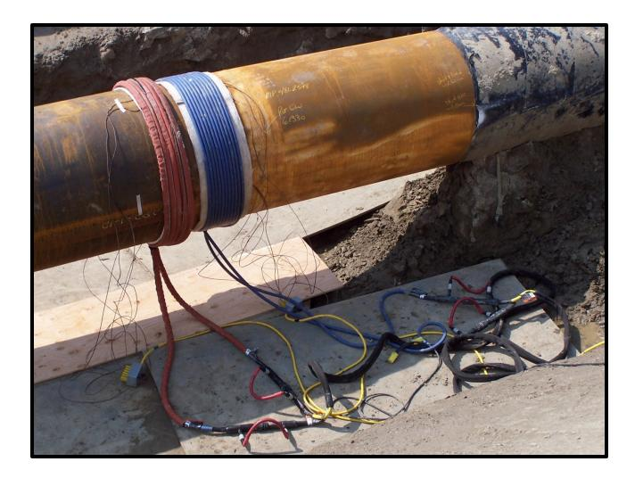
Reinforcement sleeves are commonly added to older, flowing pipelines. In this application two power sources are used to independently heat and control temperature on the parent pipe and the sleeve prior to welding.
