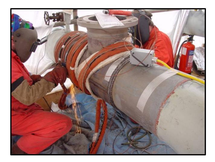
Circumferential welds are also required on each end of the split tee to secure it to the parent pipe.
