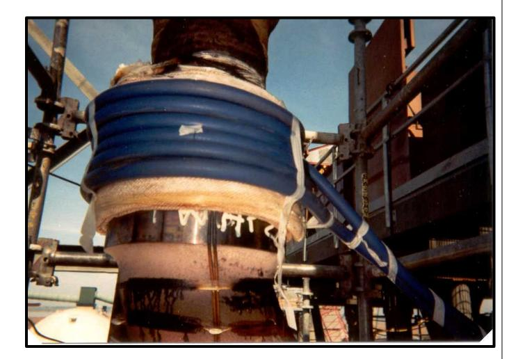
The PROHEAT is ideal for PWHT applications involving on-site welding of power plant piping subassemblies. Thermocouples are attached to the pipe according to procedure then covered with reusable woven silica PWHT insulation. The coil is then wound around the outside of the insulation, easily staying in position, even on vertical pipe.
