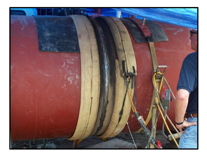
A large diameter gas transmission pipeline requires minimum interpass preheat maintenance while welding. In this application, the thermocouples are located underneath the blanket and the PROHEAT is programmed for a temperature above the minimum requirement to ensure the weld zone reaches the desired temperature.
