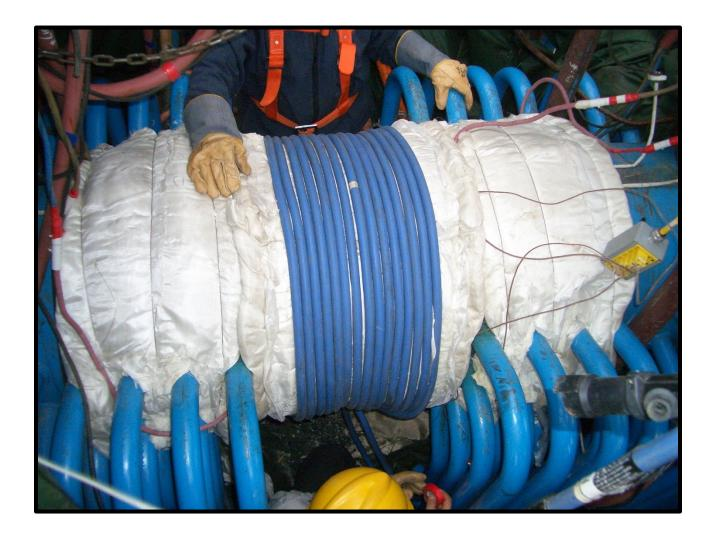
Most procedures for PWHT of P91 and P92 power plant piping call for 1400 F. (760 C) degrees for a soak temperature target. It is very important to minimize heat loss by adding insulation on both sides of the coil to retain heat.
