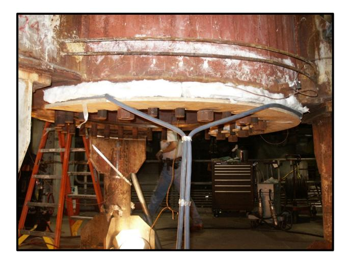
This is the installation of the coil shown in the previous application photo which was sent by the customer stating it is NOT WORKING WELL. In this application, the customer decided to use thick KAOWOOL instead of our woven silica preheat insulation. This coil was about 3" (76 mm) away from the steel, which reduced the magnetic coupling and the KW into the steel.
