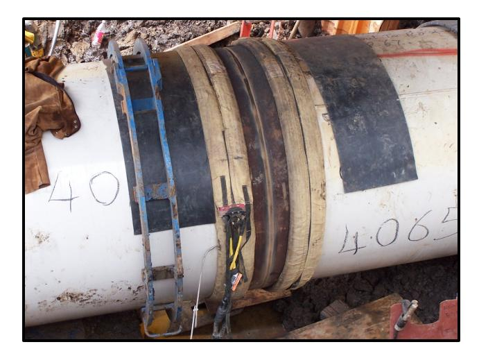
Tie-in welds requiring preheat are common during new pipeline construction. They typically take place in the trench at road bore and river crossing locations. A 75 ft. (24 m) output cable is now available to reach the pipe far from the trench. The external line-up clamp shown to the left of one of the coils was in position for the tack welds, and then moved off to the side to complete the weld.
