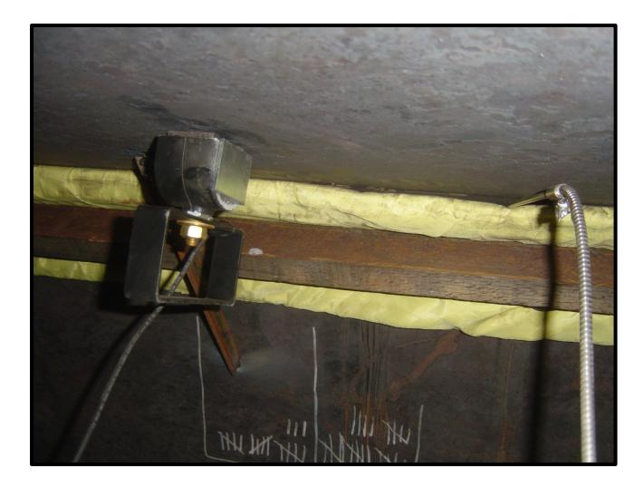
Thick, structural plates often require preheat prior to welding. In this application, the steel plate is being preheated from the opposite side of the plate. A long wood board is used to press the induction heating blanket against the steel. Control thermocouples are always positioned on the coil side of the steel as shown (TC probe on the right).
