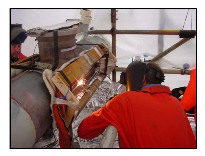
A split tee is being welded to a flowing refinery pipe (hot tap). Localized preheat is easily done with induction heating to maintain interpass temperatures while welding. A wood fixture is being used to hold the coil along the seam weld joining the two sections.
