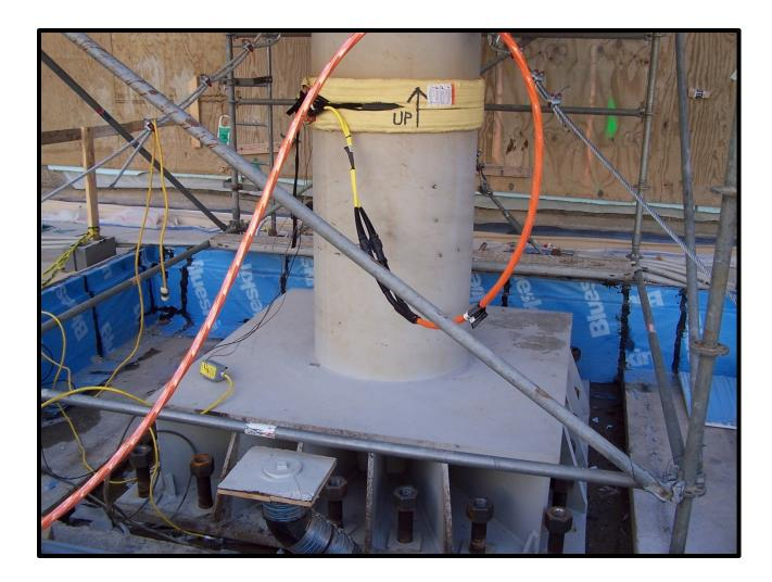
Heavy wall pipe is sometimes used as structural support beams for overhead structures. These might include offshore platforms, building pilings, or roofs, as in this case. Many welding procedures for these require preheat to minimize risks of hydrogen cracking in the weld. Note that the blanket stays in position on a vertical pipe.
