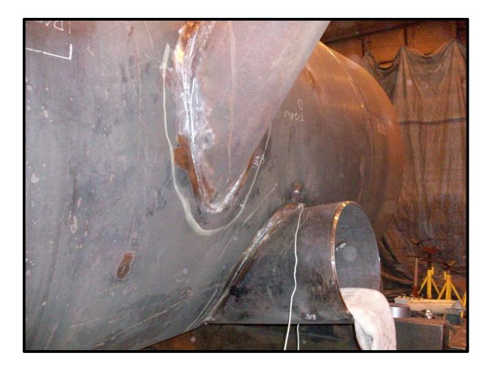
The coil fixture in the previous picture will slide into the ID of the angled branch connection to preheat the pipe from the inside out. The fixture has a diameter less than the ID of the pipe segment to allow room for preheat insulation to protect the coil.
