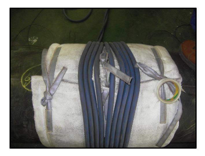
Coils can be easily spread apart to balance temperatures if needed. In this application, the small diameter weldolet shown in the previous photo is covered by the PWHT insulation and the coils are slightly flared apart to uniformly heat around it.
